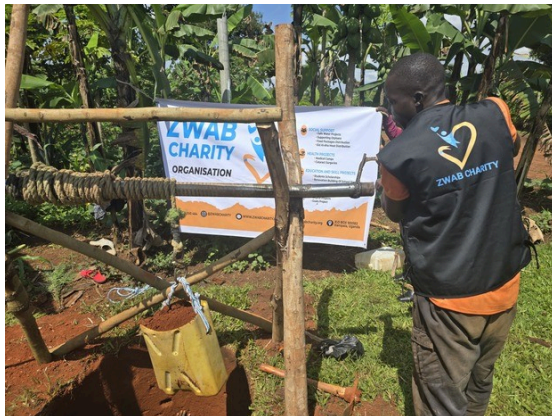
A Zwab team member stands beside an excavated opening.
